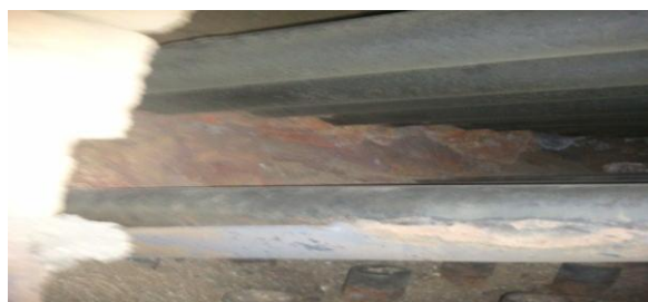
Fig.3 combustion chamber of boiler
